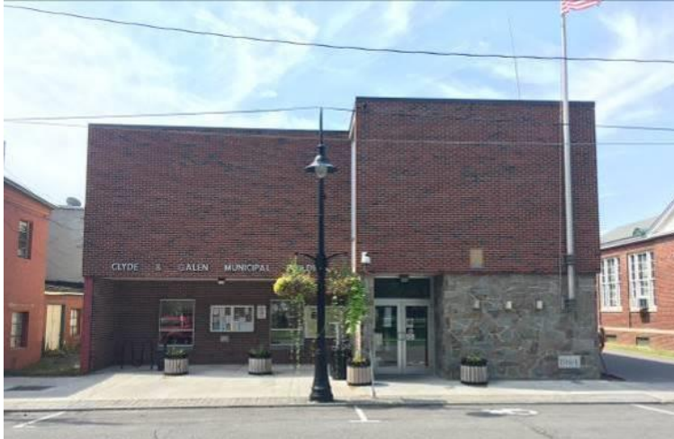
Photo 2- 14: 6 S Park Street; Town of Galen Municipal Building
